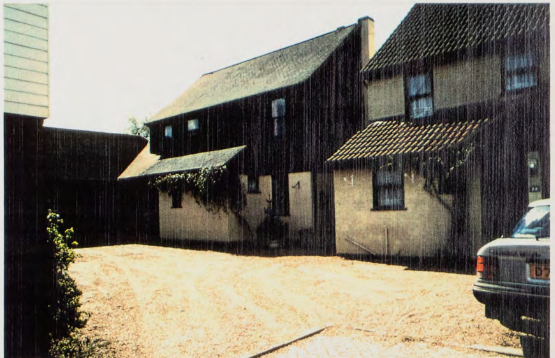
The cul de sac off the entry is gravel and is maintained by the owners. The grouping of buildings is quite urban and fits in with the surrounding village of Ingatestone, a small historic village.
