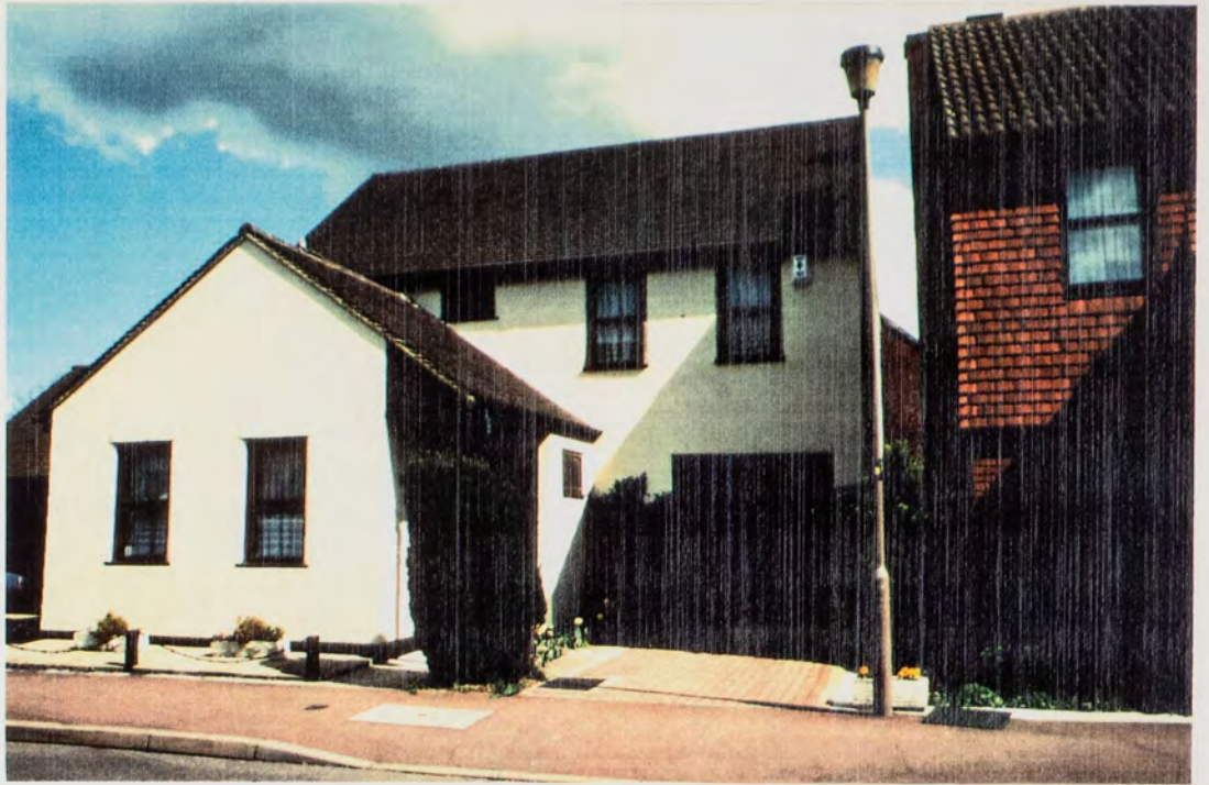
Garages are incorporated into the house itself in some places. This solution is only possible in two storey houses when higher densities are to be maintained without excessive ground cover.
