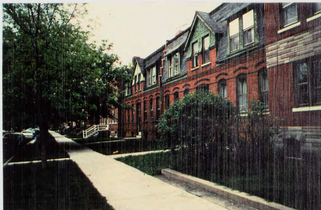
The workers' housing was solidly constructed of brick with slate roofs. Backyards are connected to rear service lanes.
